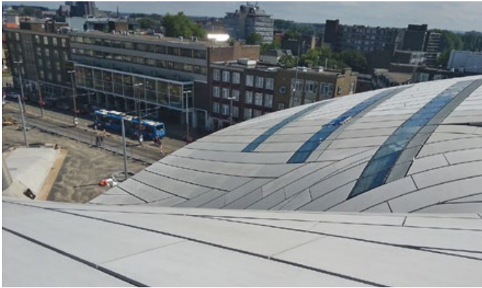
This view of the roof shows the tolerances the precast fabricator was able to achieve using the reconfigurable mould.
