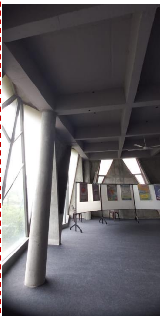
Figure 5.2.3 – slant columns and waffle slab
