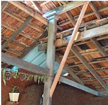
Detail of the corner rafter and column.
