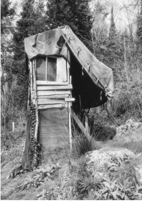
10.15 The compost toilet. The small sign with its arrow directs users to the entrance up the flight of steps. The collection chamber below is protected from flies by mesh screening.
