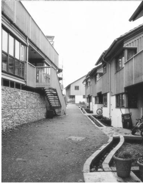
10.4 Main Street. This illustration also shows the drainage rills for surface water, part of the SUDS system.
