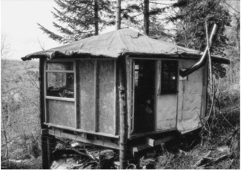
10.11 A hexagonal bender, incorporating the use of sterling board. This dwelling has a panoramic view across the valley to the Devon hills.
