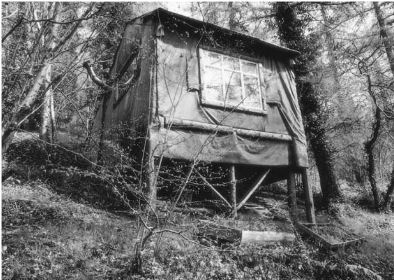
10.10 One of the benders, also constructed of timber and tarpaulin. The twisted chimney from the wood burning stove can be seen on the left.
