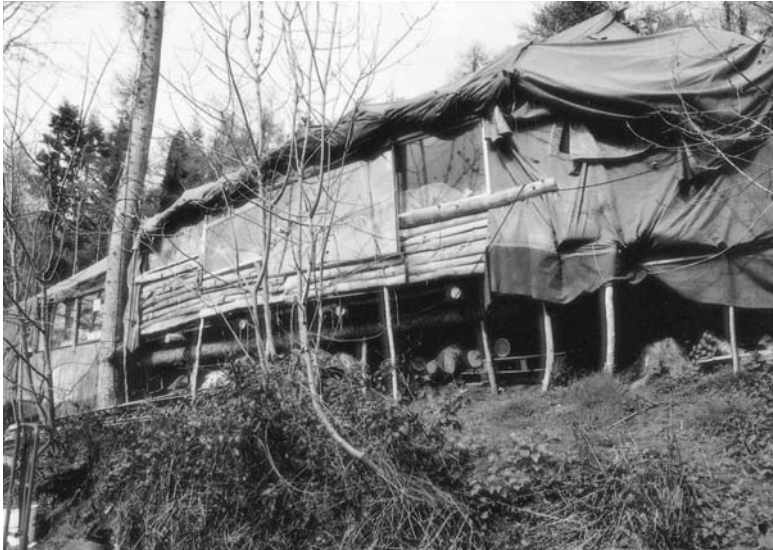
10.9 The communal longhouse made from wood, recycled windows, and tarpaulin. The cantilevered construction provides extra storage space.
